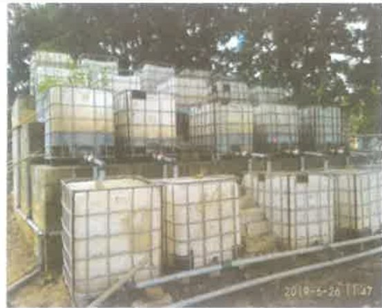
Fig. 5 5kld Phyto-remediation system
