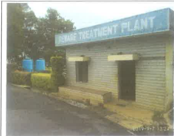
Fig. 4 Sewage Treatment Plant
